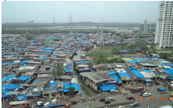
Encroached Shastri Nagar Nalla, Goregaon (W)
