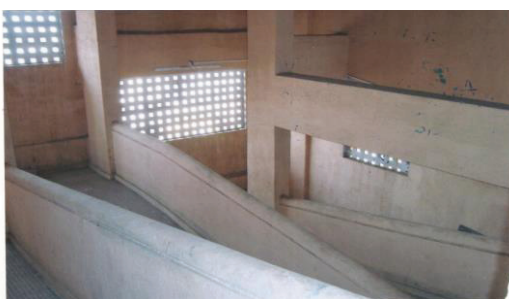
Photograph showing ramp in addition to lift and staircase
